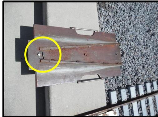
Hole is for pin that holds the transfer plate in place while moving equipment.
